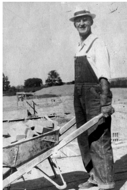
Pastor John DeWaard helping with construction of new building in Cedar Grove, Wisconsin, in the 1930s
